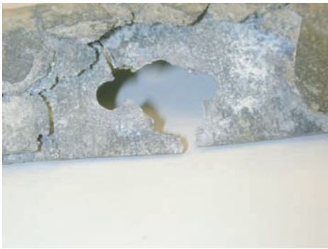
Fig. 11 Exfoliation corrosion of an aluminum T-45 cockpit kick plate angle resulting from water intrusion within cockpit areas. Courtesy of J. Benfer, Naval Air Depot, Jacksonville. See the article "U.S. Navy Aircraft Corrosion" in this Volume.
