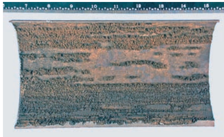
Fig. 37 Inside of a pipe in the petroleum industry exhibits mesa corrosion. Note profile of pipe wall in lower right corner. Characteristic appearance of mesa corrosion resulting from CO 2 , water, and flow. The scale is in inches. Source: InterCorr International, Inc., Houston, TX. See the article "Corrosion in Petroleum Production Operations" in this Volume.
