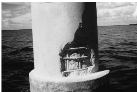
Fig. 45 Directly applied thermal-sprayed zinc sacrificial cathodic protection system protecting both exposed and embedded reinforcement
