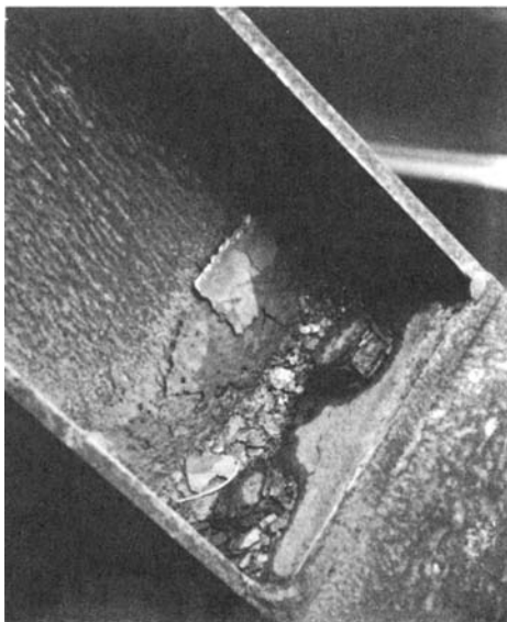
Fig. 11 Heavy corrosion scale buildup on structural members of weathering steel at a pocket where water could collect and stand
