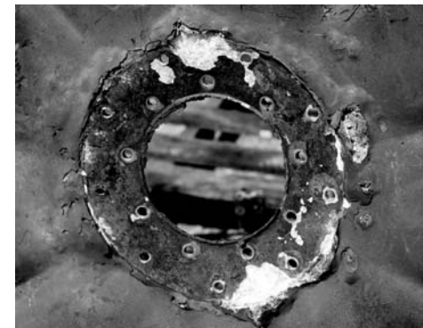
Fig. 7 Firing platform exfoliation corrosion. Source: Ref 5
