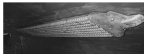
Fig. 5 Keel heat exchanger installation
