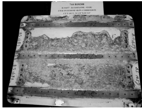
Fig. 6 Corrosion of 747-400 interior 2024-T351 aluminum belly skin machined interior aluminum cladding
