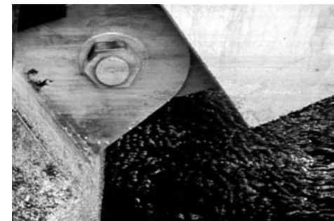
Fig. 30 Stainless steel arch hinge. Note marine growth
