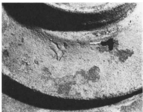
Fig. 3 Uniform corrosion of ACI CD-4MCu cast stainless steel pump impeller after 1 year in an environment containing 50% H_3PO_4 and 10% gypsum. Courtesy of A.R. Wilfley & Sons, Inc., Pump Division
