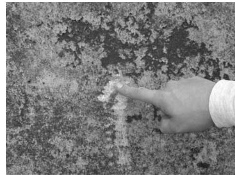
Fig. 48 Cement paste losses due to liquid-phase carbonation in a pure oxygen reactor for a pulp and paper mill
