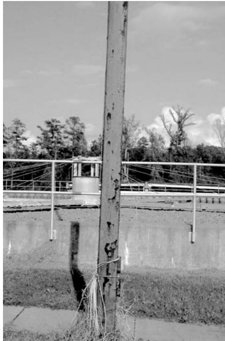
Fig. 1 Corroded low-carbon steel light pole due to corrosive atmosphere at a wastewater treatment plant on a military installation
