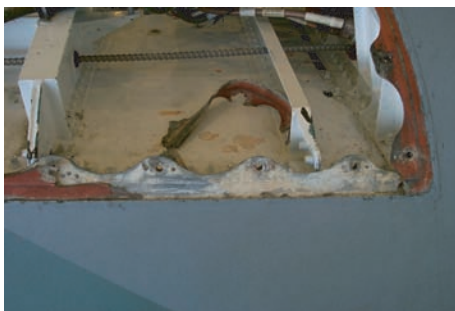
Fig. 13 Galvanic corrosion of F/A-18 aircraft dorsal scallops resulting from composite doors attached to aluminum substructure with titanium and steel fasteners in the presence of moisture. Courtesy of S. Long, Naval Air Depot, North Island. See the article "U.S. Navy Aircraft Corrosion" in this Volume.
