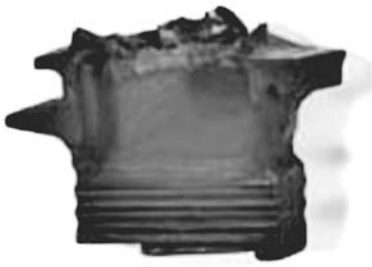
Fig. 7 Failed shipboard turbine at the transition between blade and stem. See also Fig. 8 through 11.
